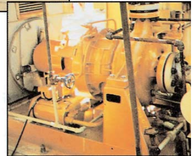
Full emission BMP-338 (500 gpm at 1000 feet) hydrocarbon bottoms pump
